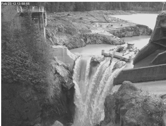
Glines Canyon Dam Removal National Park Service
